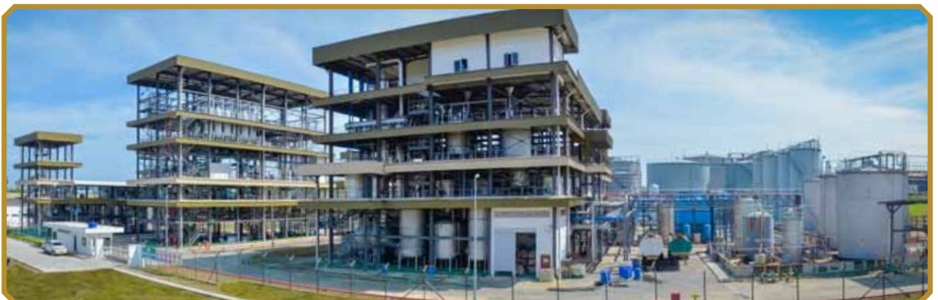
Overview of SOP Green Energy plant complex
